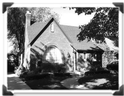
1753 Period Revival | English Cottage Built 1929
