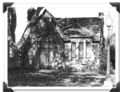
1759 Period Revival | English Cottage Built 1929
