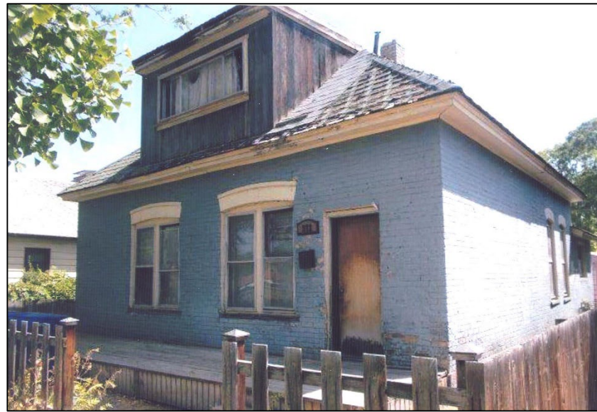
single family residence – before
